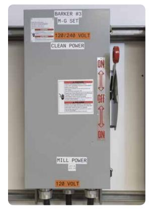
Figure 10: Electrical boxes or panels should be labelled or marked to indicate the machine, equipment, or process supplied and the energy type and magnitude.
