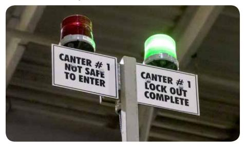
Figure 6: An indicator showing that it is safe to enter the area.
