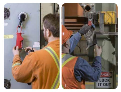
Figure 13: (A) A worker applying locks. (B) A worker applying a restraint pin.
