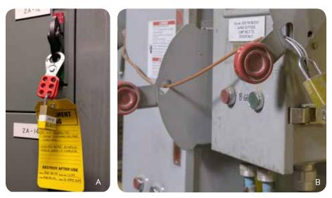
Figure 14: (A) A lock with a tag. (B) A cable lockout.
