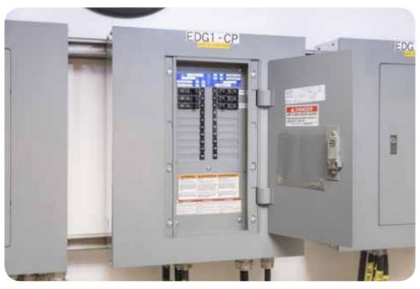
Figure 8: Main power panels — circuit breaker panel.
