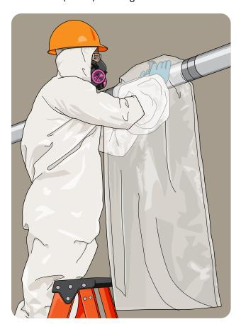
A worker uses a glove bag to remove asbestoscontaining pipe insulation.
