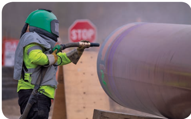
A worker sandblasts a pipe joint before welding.
