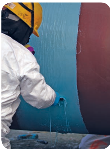
Coating the inside and outside of pipes helps prevent corrosion from groundwater or product contaminants.
