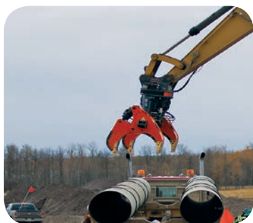
Lifting clamps must be certified and compatible with the equipment they are attached to.
