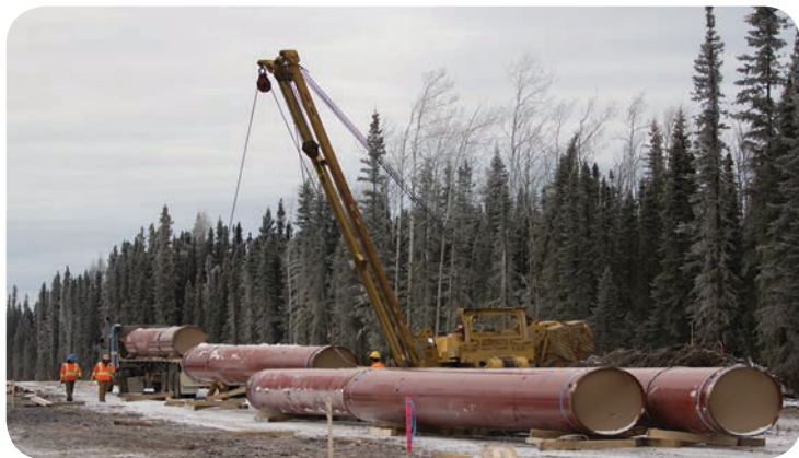
A side boom unloads large-diameter pipe from a truck at a delivery point along the ROW.
