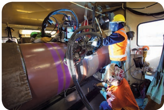
Workers monitoring automatic welders inside portable welding shacks are at risk of exposure to a hazardous atmosphere. There must be an ECP and suitable ventilation.
