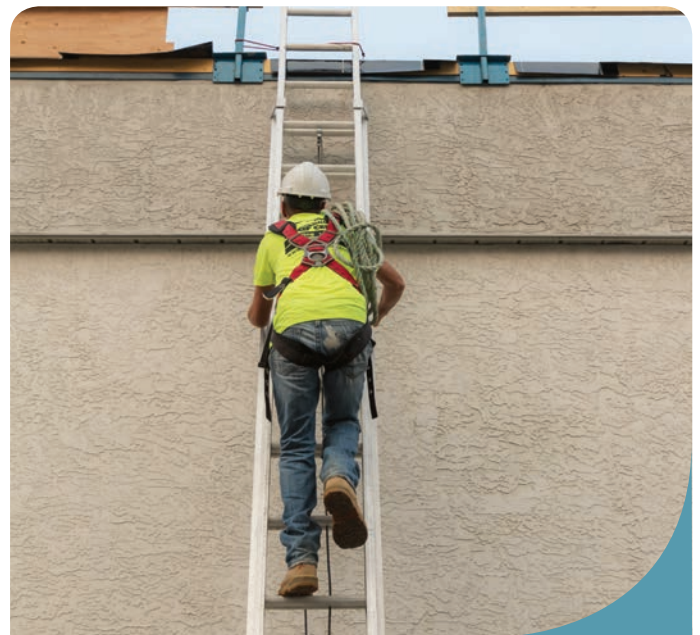
Dennis Johnson from the Roof Doctor using three points of contact.
