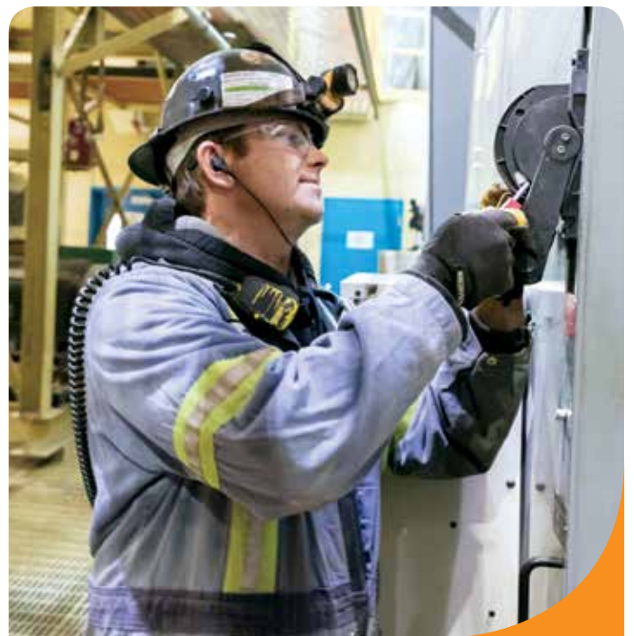
Demonstrating a lockout procedure at Pinnacle Renewable Energy's Meadowbank/Hixon pellet plant.
