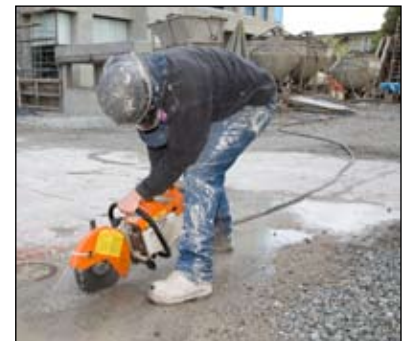
Worker cutting concrete using water for dust control
