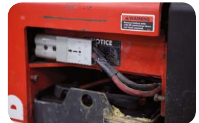
Inspect cables for damage
