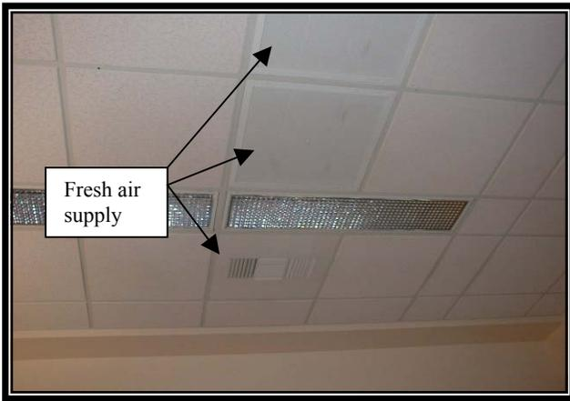
Plate 7: View of fresh air supply located in the ceiling of the labour and delivery room.
