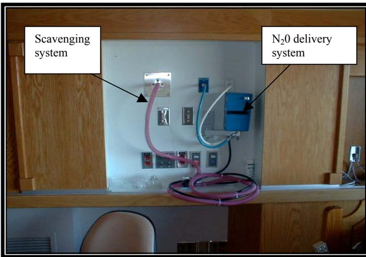
Plate 5: View of nitrous oxide delivery system and scavenging system.
