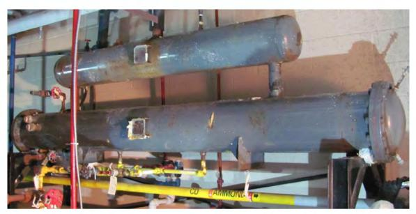
Figure 18: The curling rink chiller with the insulated cladding removed.
