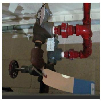
*Figure 17: The pressure-relief manifold installed on top of the surge tank for the curling rink* chiller.
