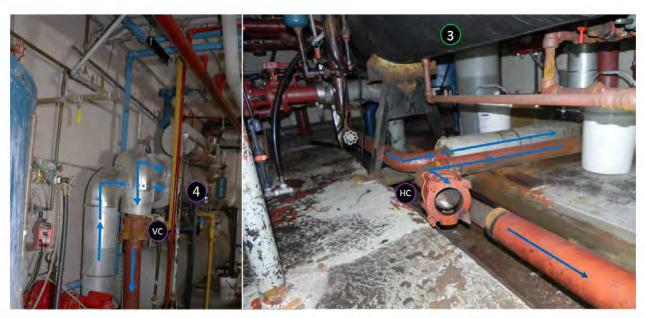
**Figure 13:** The photograph on the left shows the position of the vertical coupling (VC) on the brine outlet pipe of the curling rink chiller (4). The photograph on the right shows the horizontal coupling (HC) under the hockey rink chiller (3) and downstream of the VC. The normal brine circulation path is indicated by the blue arrows.
