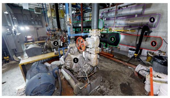
*Figure 3:* The compressor room, looking east, showing compressor 1 (1), compressor 2 (2), the hockey rink chiller (3 - green outline), the curling rink chiller (4 - purple outline), and the receiver (5 - red outline).
