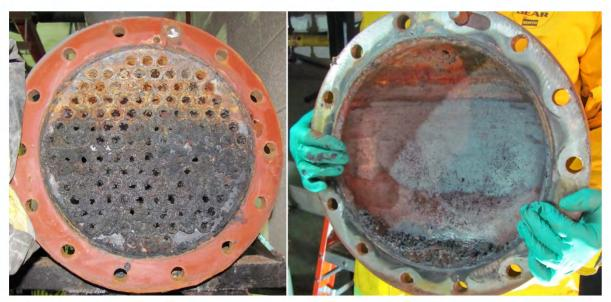
*Figure 20:* The photograph on the left shows the return end of the tube sheet of the curling rink chiller with the gaskets intact. The photograph on the right shows the return end dome cover.
