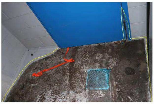
*Figure 10:* Vestibule floor and door. The oily liquid flowed under the door and through the hinge area. The blue colour on the brass floor plate indicates exposure to ammonia.
