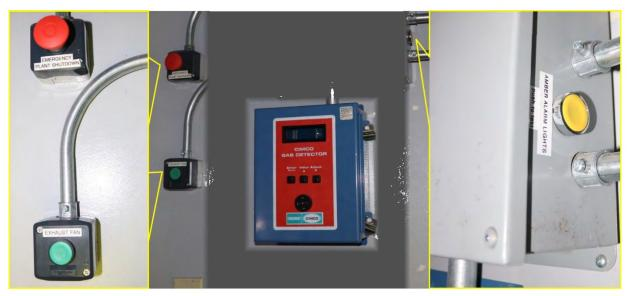
*Figure 8:* Composite image showing the ammonia gas detector system located in the vestibule outside of the compressor room.
