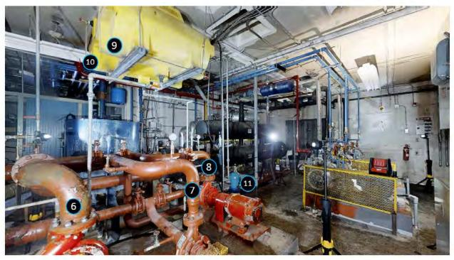
*Figure 4:* The compressor room, looking south, showing the hockey rink brine pump (6), the auxiliary brine pump (7), the curling rink brine pump (8), the hockey rink brine expansion tank (9), the curling rink brine expansion tank (10), and the curling rink brine filter (11). The hockey rink brine filter is not shown.
