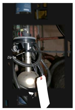
*Figure 16:* Photograph showing a black plastic zip tie used to defeat the factory setting on the ammonia liquid high-level shutdown switch on the hockey rink chiller.
