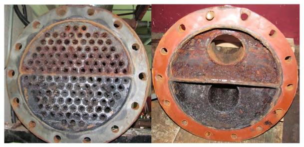
*Figure 19:* The photograph on the left shows the inlet/outlet end of the tube sheet of the curling rink chiller. The photograph on the right shows the dome cover with gasket in place as intended.
