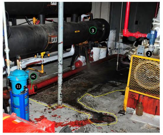
**Figure 9:** The compressor room, looking southeast, showing the brine outlet pipe that separated at HC (horizontal coupling), located under the hockey rink chiller (3). The black, oily liquid that sprayed out of the separated pipe is outlined by the dotted yellow line. Also shown are compressor 2 (2) and the curling rink brine filter (11). (Orange paint is visible through the top coat of grey paint on the concrete floor.) (Source: Ram Environmental Response Ltd.)
