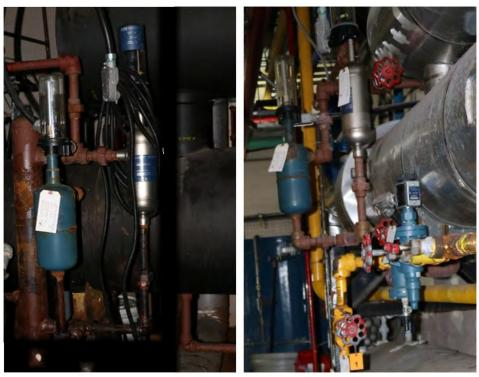
*Figure 7:* The photograph on the left shows the hockey rink chiller liquid level control (blue tank) and the ammonia liquid high-level shutdown switch (silver tank). The photograph on the right shows the same control and switch on the curling rink chiller.
