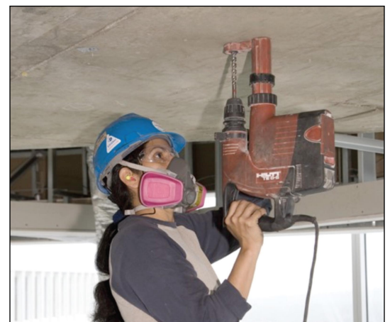
Concrete drill with a HEPA filter attachment.
