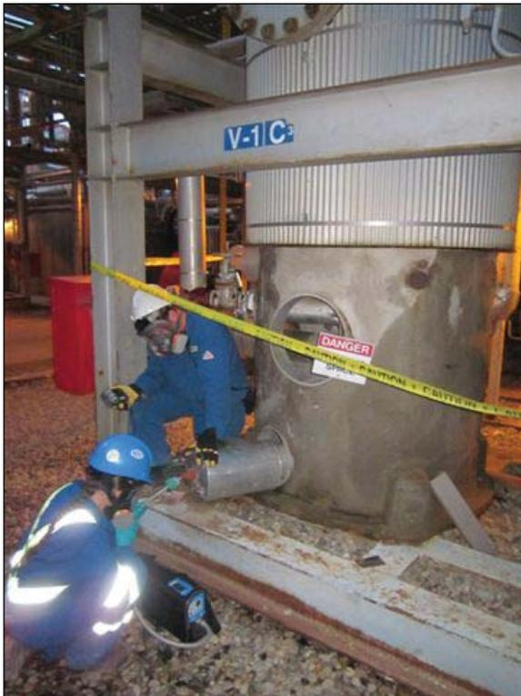
*Workers wear respirators while testing for mercury*
