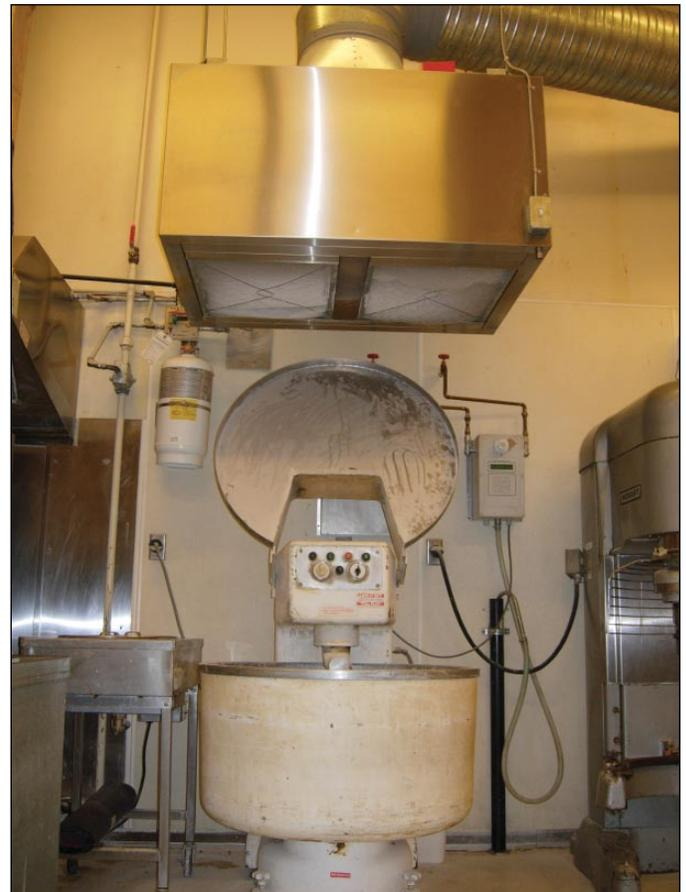
*Dough mixer retrofitted with a cover and exhaust ventilation*
