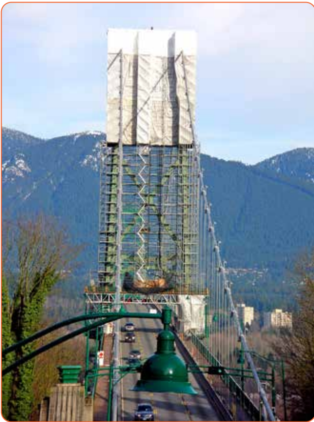
Containment of a lead removal operation on a bridge
