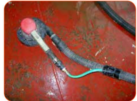
Grinder with a HEPA exhaust attachment
