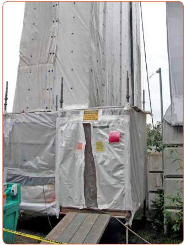
Entrance to a lead removal enclosure
