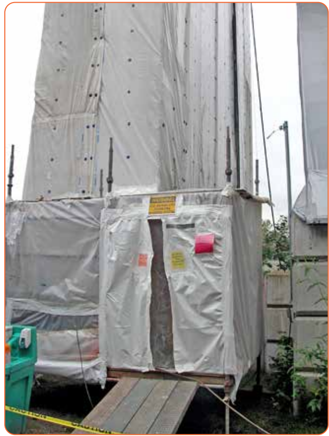
Entrance to a lead removal enclosure
