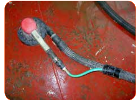
Grinder with a HEPA exhaust attachment
