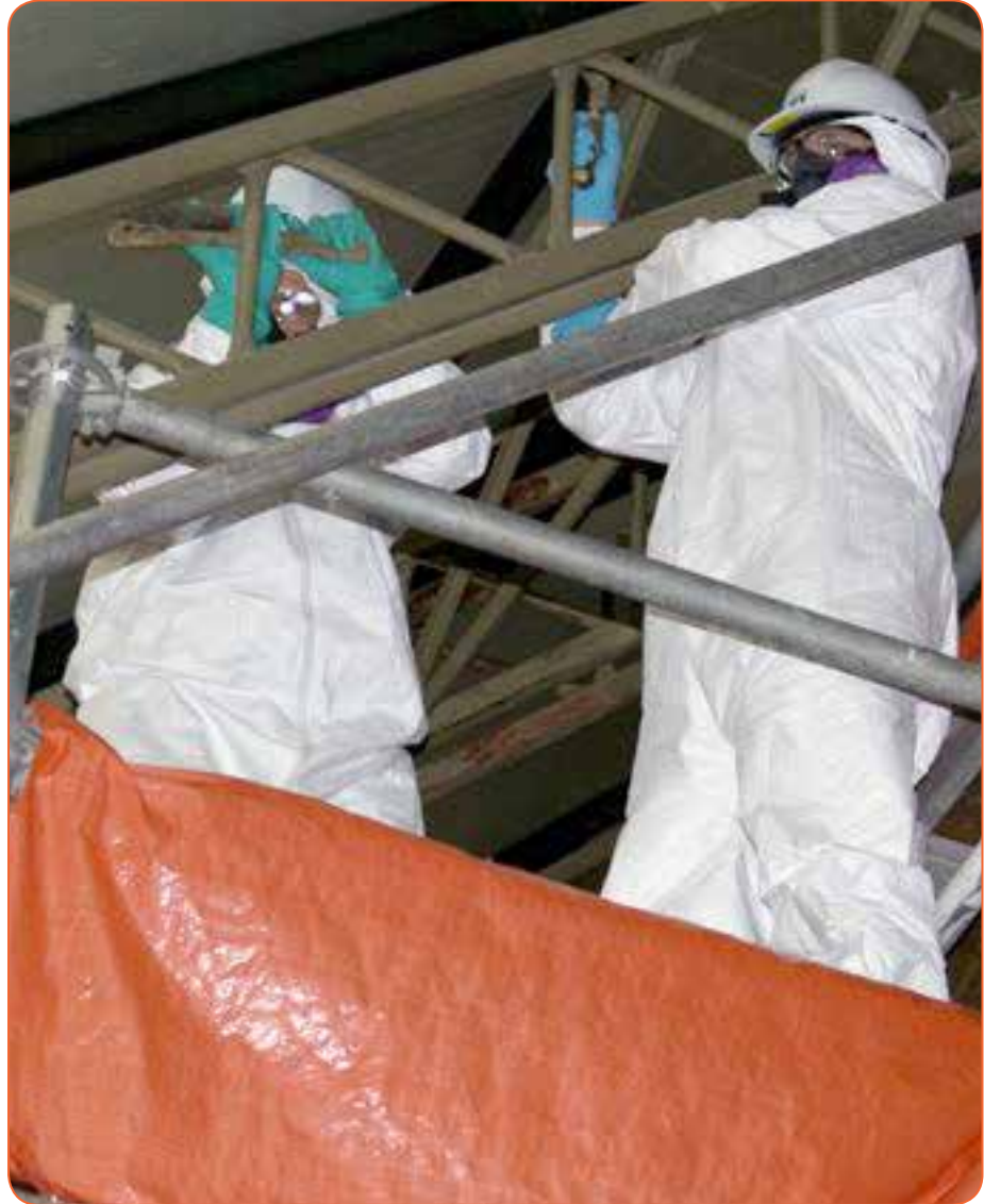
Workers hand-brushing lead residue from a steel structure
