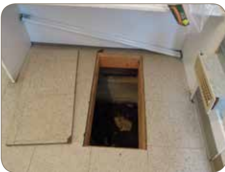
Interior crawl space entrance
