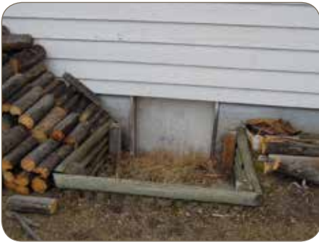
Exterior crawl space entrance
