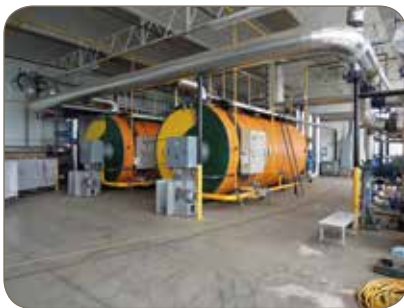
Gas-fired boilers
