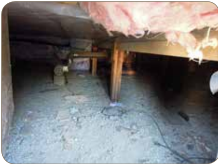
Exterior entrance and crawl space
