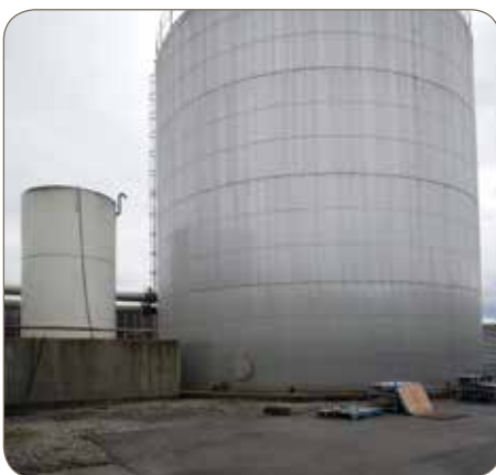
Closed steel tanks
