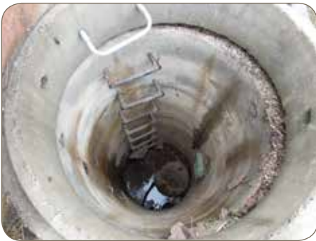
Stormwater manhole
