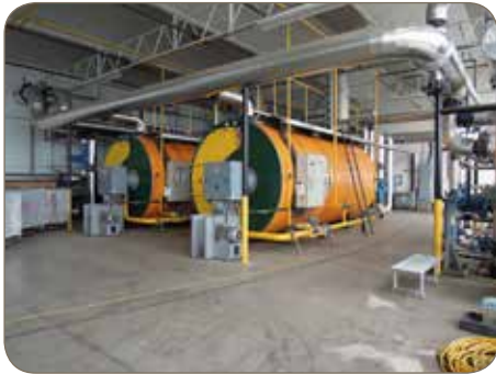
Gas-fired boilers
