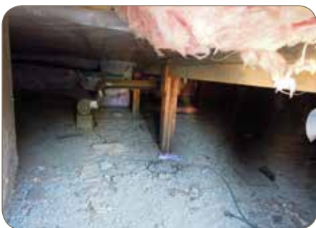
Exterior entrance and crawl space
