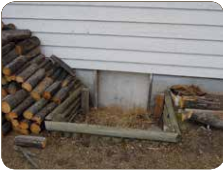
Exterior crawl space entrance
