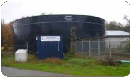
Above-ground manure tank
