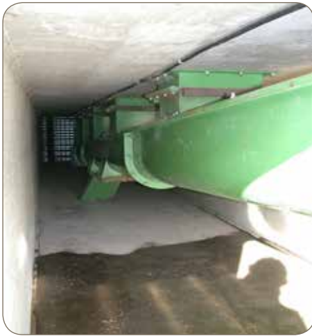
Conveyor in a tunnel
