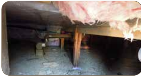
Exterior entrance and crawl space
