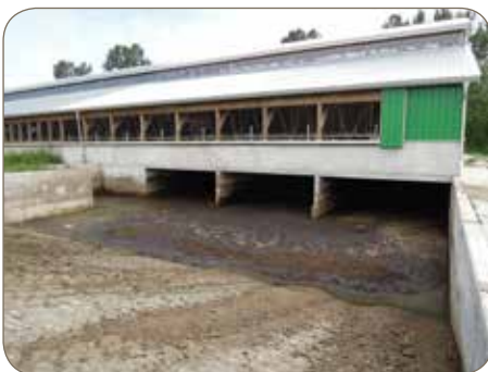
Subfloor manure storage
