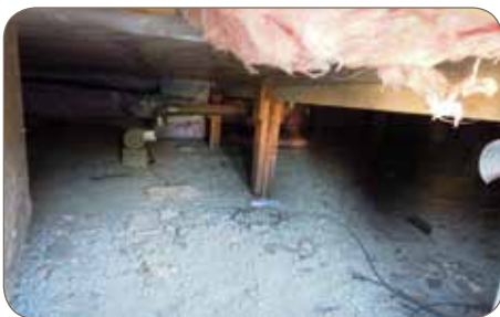
Exterior entrance and crawl space
