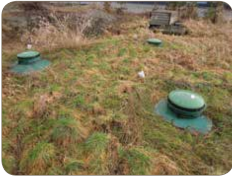
Septic tank hatches
