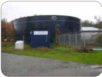
Above-ground manure tank
