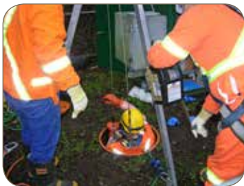
Worker entering a manhole
