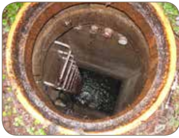
Sanitary sewer manhole
