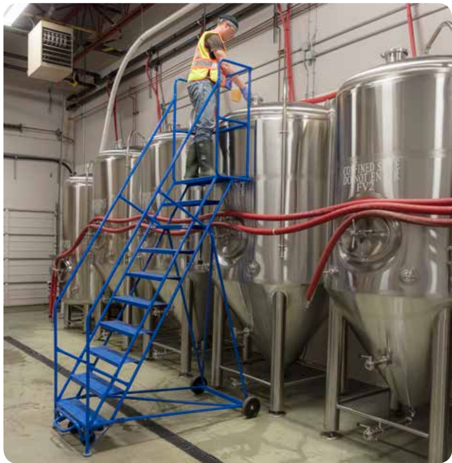
Platform ladders allow workers to perform tasks safely at the top of tanks.
