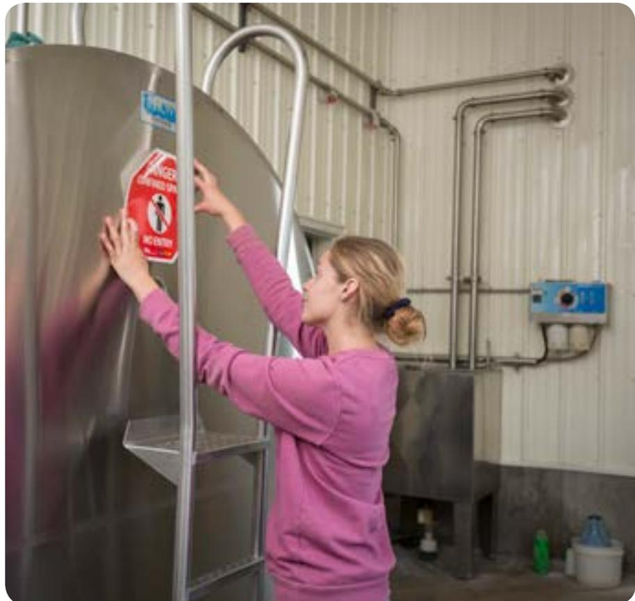
Confined spaces should be marked with appropriate, visible signage warning workers of the hazard.
