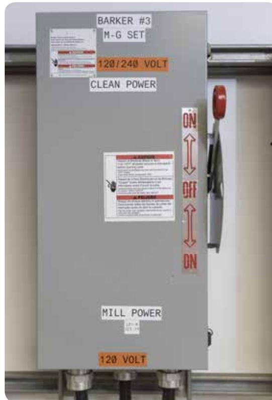
Figure 10: Electrical boxes or panels should be labelled or marked to indicate the machine, equipment, or process supplied and the energy type and magnitude.
