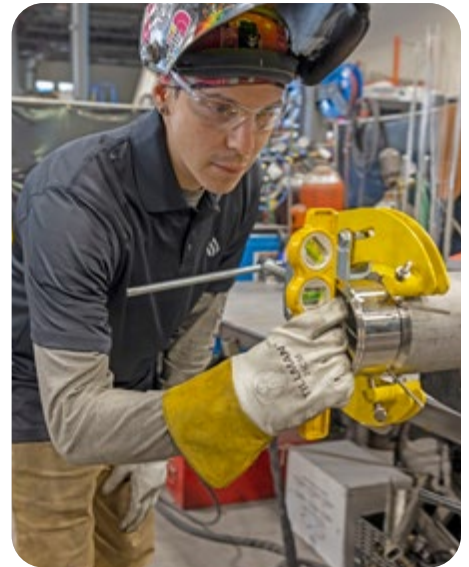
Vitalis employee Justin Peters leveling an extractor pipe before welding.
