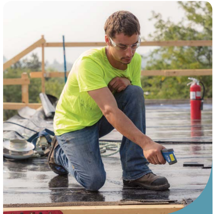
Mike Francis recording temperatures using an infrared thermometer.
