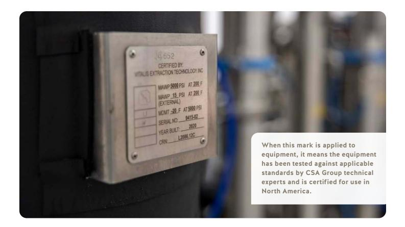
permit, and sign off on pressurized equipment. Once it's approved for use, a CSA label is applied.
