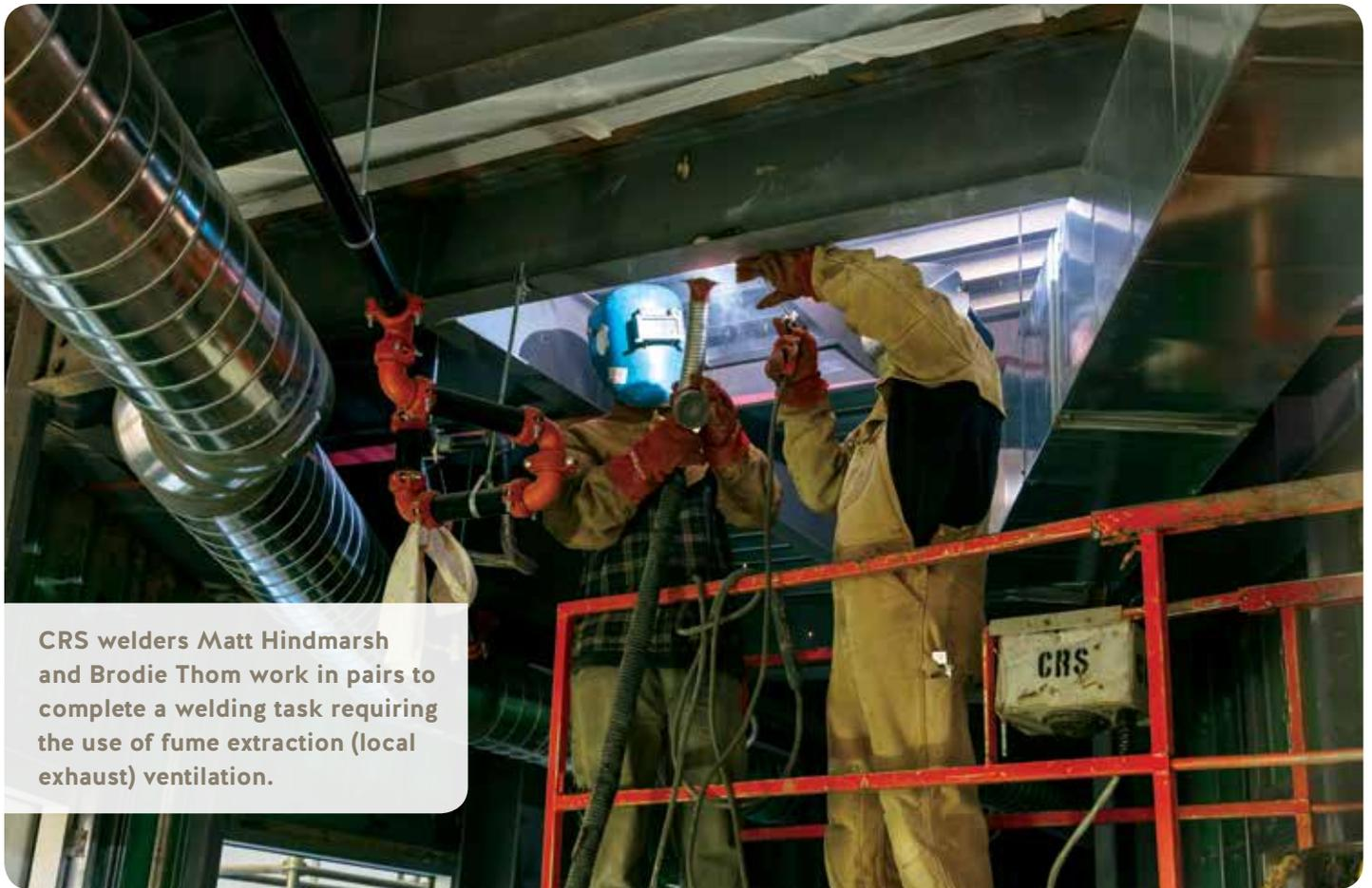
CRS welders Matt Hindmarsh and Brodie Thom work in pairs to complete a welding task requiring the use of fume extraction (local exhaust) ventilation.
