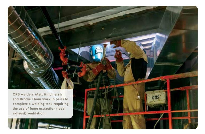
"Substituting a lower alloy electrode or wire can make a significant reduction in fume generation," says Jopling. "The selection of substitutes is complex as many variables and certifications need to be considered."
