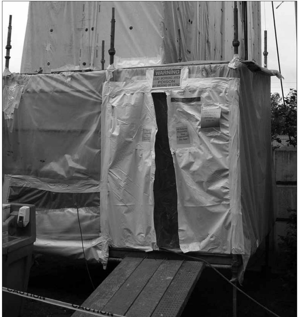
Entrance enclosure for lead removal
