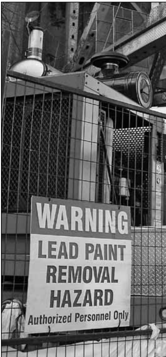
Warning sign on a lead removal site
