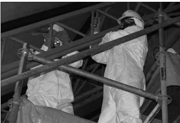
Workers hand-brushing lead residue from a steel structure
