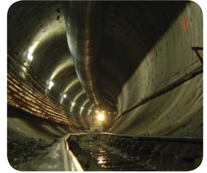
Bored Tunnel Construction
