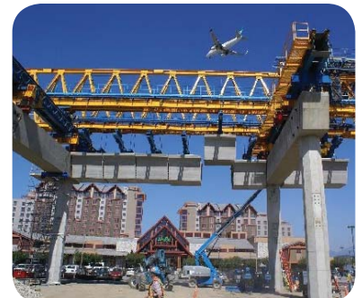
Elevated Guideway Construction
