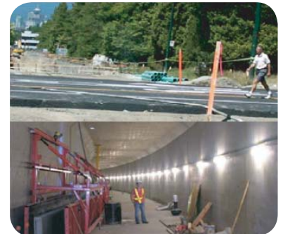
Cut-and-Cover Tunnel Construction
