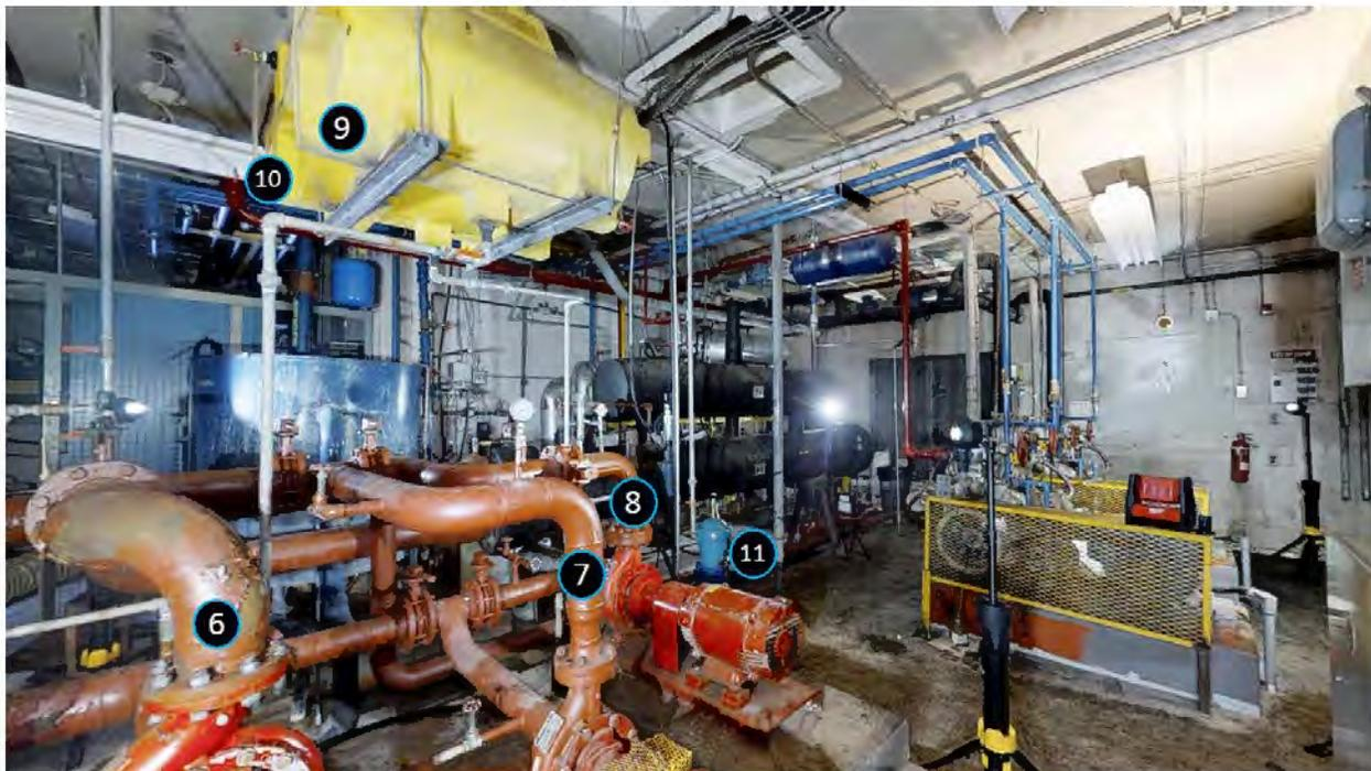
**Figure 4:** The compressor room, looking south, showing the hockey rink brine pump (6), the auxiliary brine pump (7), the curling rink brine pump (8), the hockey rink brine expansion tank (9), the curling rink brine expansion tank (10), and the curling rink brine filter (11). The hockey rink brine filter is not shown.
