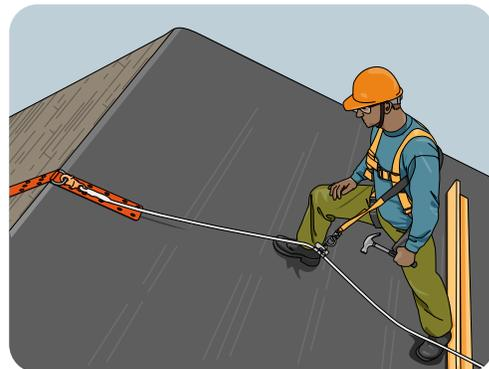
Left: A synthetic webbed anchor strap and a metal roof anchor (ridge anchor). Right: Fall-restraint systems prevent workers from falling from a work position or from travelling to an unguarded edge.
