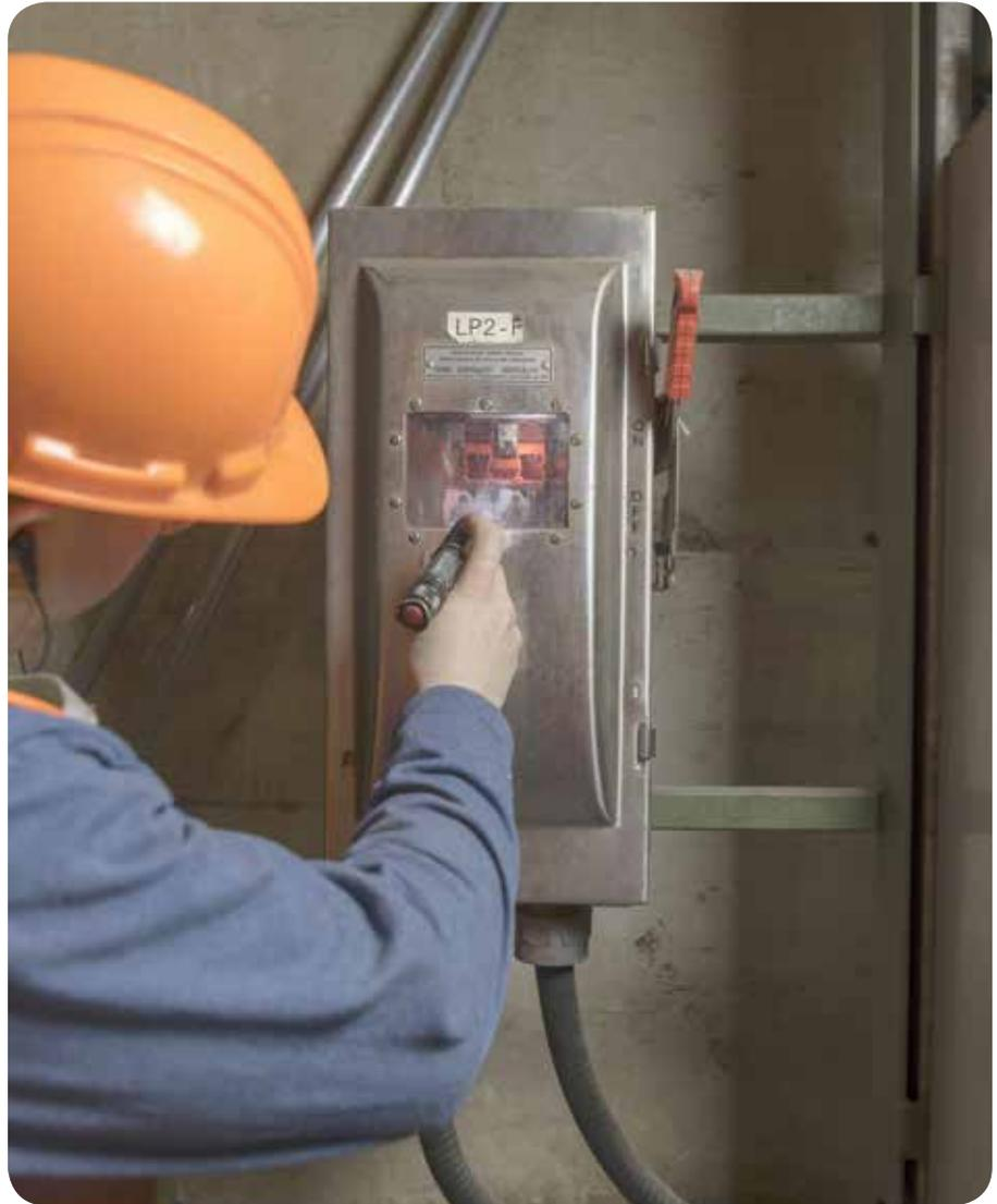
Figure 5: A worker observing the blades disengaging in a visible blade disconnect switch (visi-disconnect) panel.
