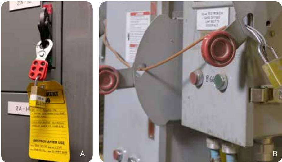
Figure 14: (A) A lock with a tag. (B) A cable lockout.
