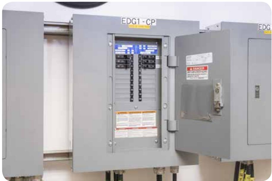
Figure 8: Main power panels — circuit breaker panel.
